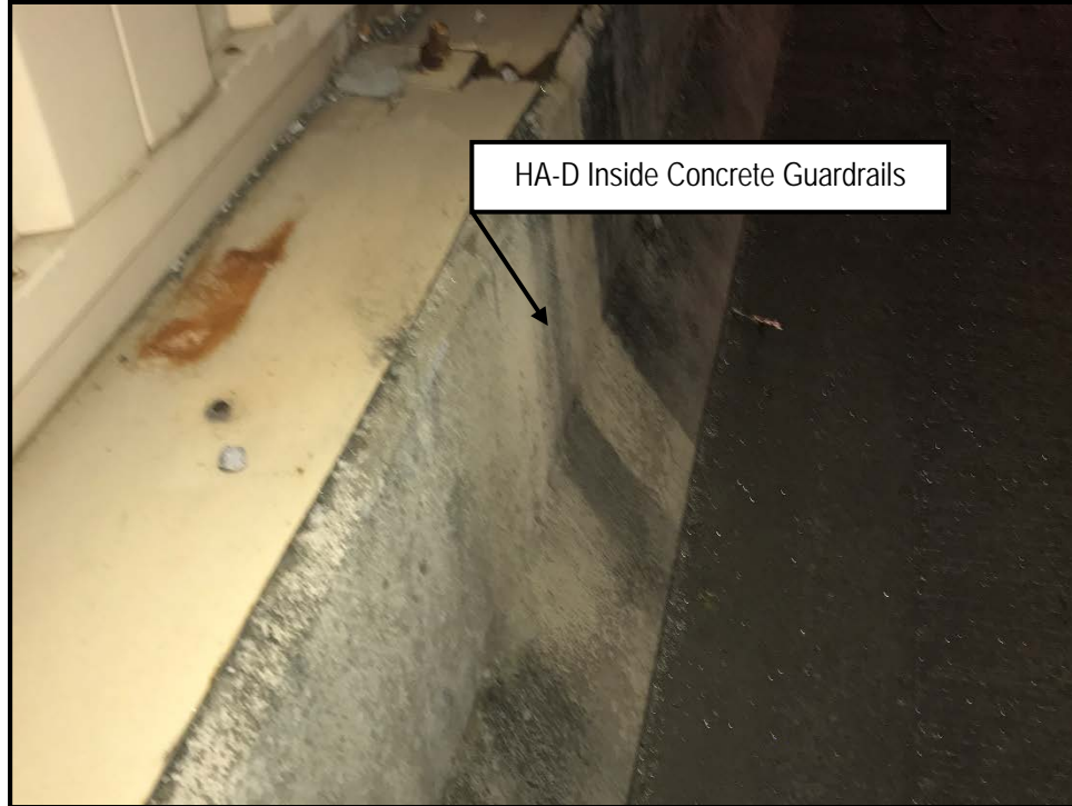
Photo 4: View of HA-D on the eastbound I-440 bridge over Craig Avenue
