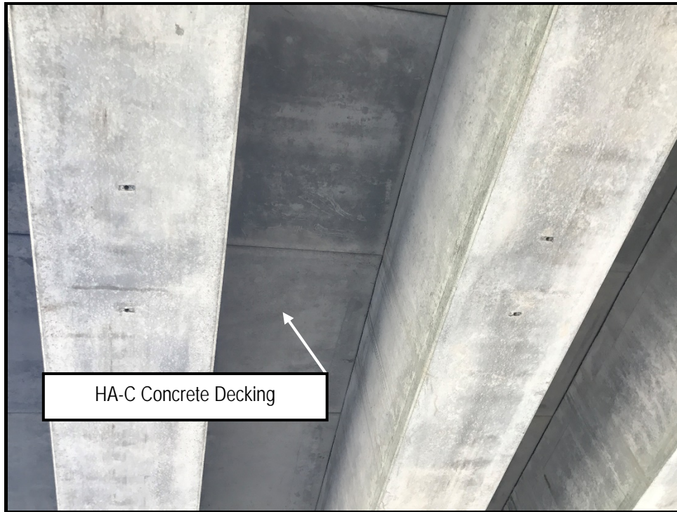
Photo 3: View of HA-C on the eastbound I-440 bridge over Craig Avenue
