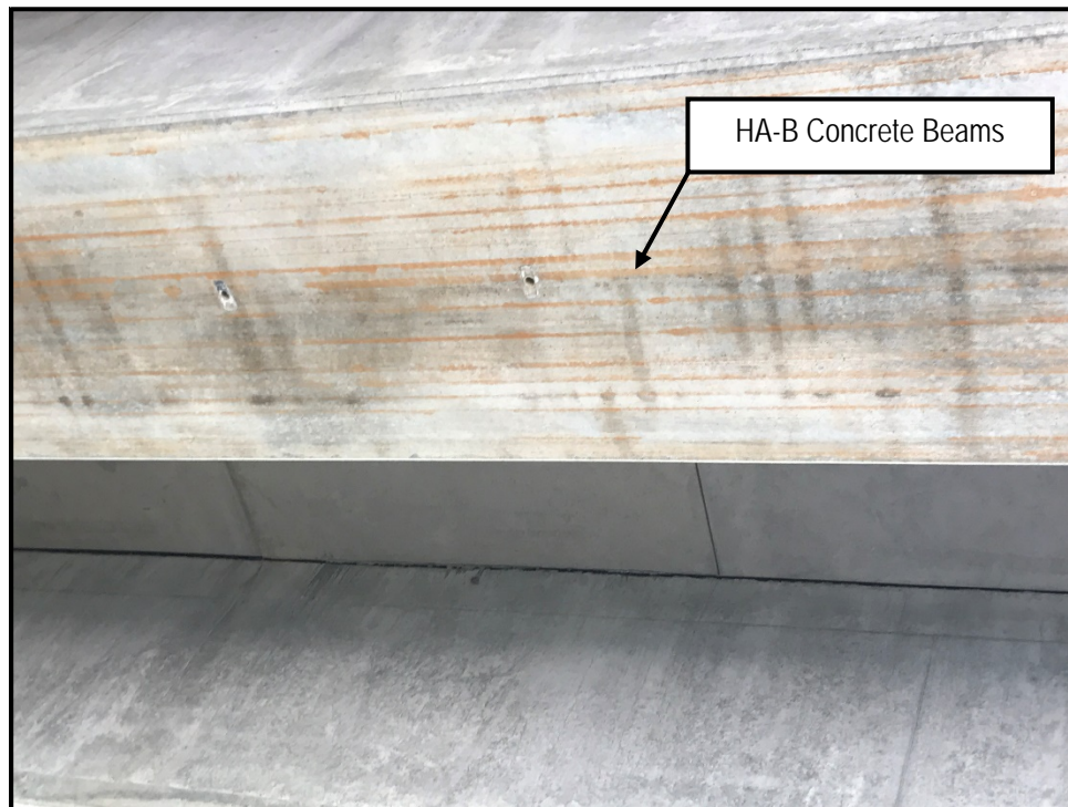
Photo 2: View of HA-B on the eastbound I-440 bridge over Craig Avenue
