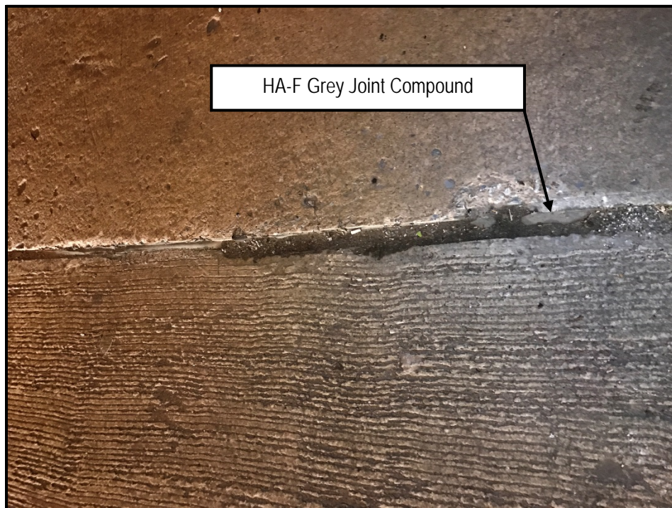
Photo 6: View of HA-F on the eastbound I-440 bridge over Craig Avenue
